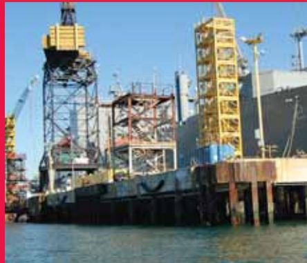
Structural Enhancement of NASSCO Berths III & IV , San Diego, USA
