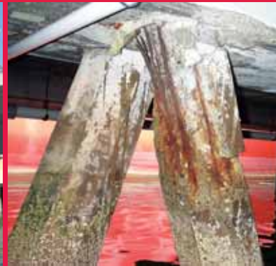
Concrete Repair and Protection on Chula Vista Bayside Park Pier , CA
