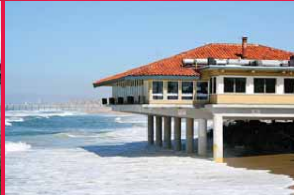
Structural rehabilitation and repair of Redondo Beach Restaurant , California
