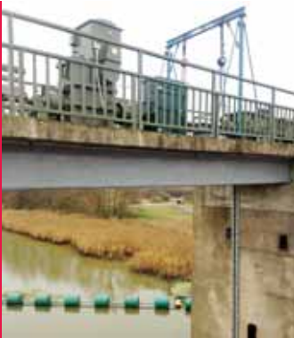
Structural Strengthening of AG Wrights Sluice Gates , Denver, Norfolk, UK
